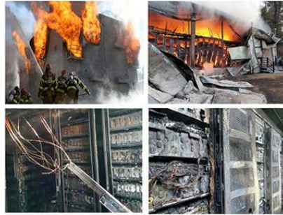
Figure 14: Fire Damage at Korean BESS Facilities 229
